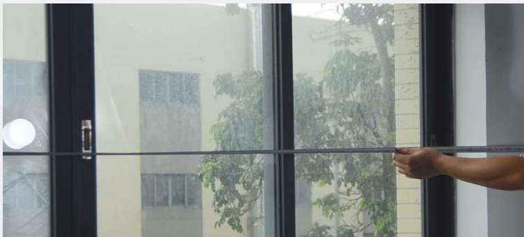
Measure the wall dimensions and confirm the installation length
